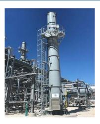
Gas Storage Facilities: Long term storage of natural gas and LNG often contain water vapor which accumulates over time, thus separators are utilized in gas storage facilities prior to being sent to a compressor station or used by customers.
