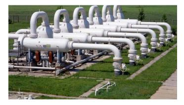
Regulator and Metering Stations: These are located strategically throughout the natural gas distribution pipeline to control flow rate and pressure. Gas/liquid separators ensure that the gas entering these stations are free from liquid contaminants, protecting expensive flow meters and improving accuracy of their measurements by separating entrained contaminants.
